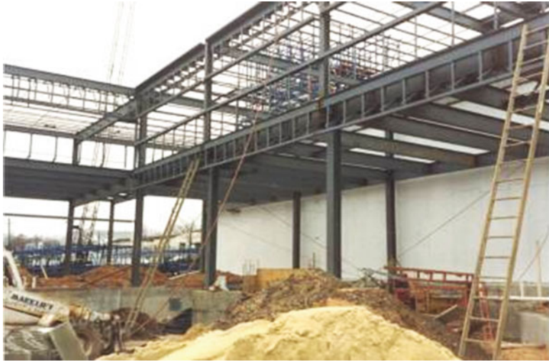
Fig. 12.5 Steel frame and brick construction
