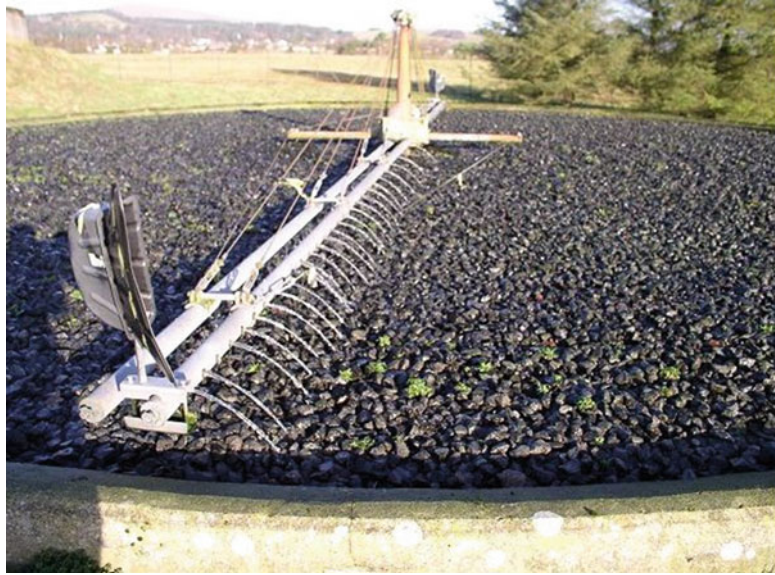
Fig. 18.8 Typical percolating (trickling) filter
